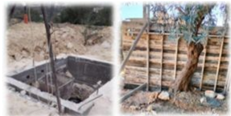
Above: new wells under construction
